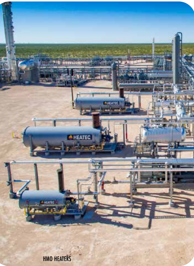
GAS REGEN HEATER AND THERMAL FLUID HEATER
