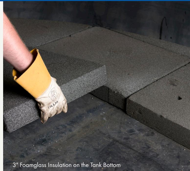
3" Foamglass Insulation on the Tank Bottom
