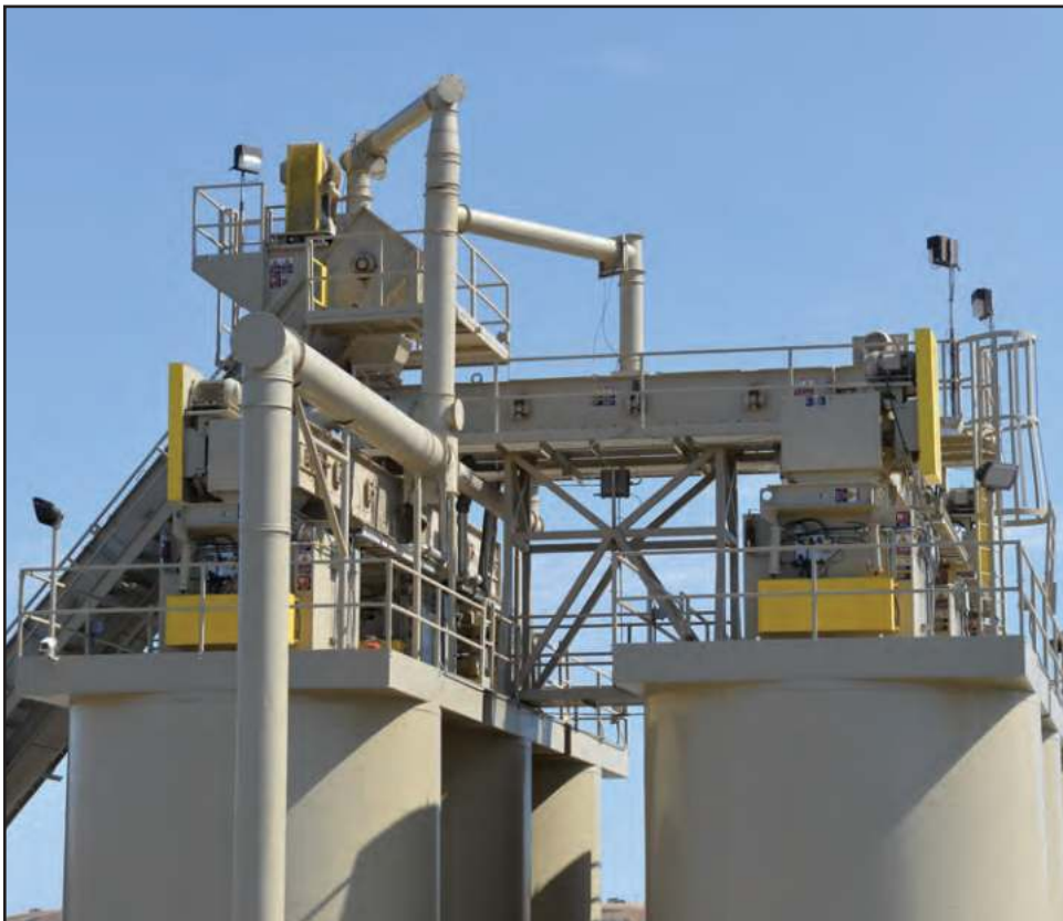
The New Generation Storage System is topped with a horizontal 36 in x 25 ft (91.44 cm x 7.62 m) crossover traverse conveyor.
