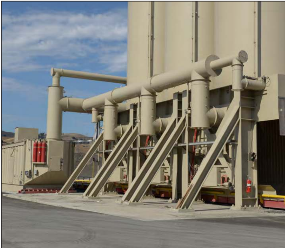
The DeSilva Gates asphalt plant is outfitted with a blue smoke system to help meet California's stringent air quality standards.
