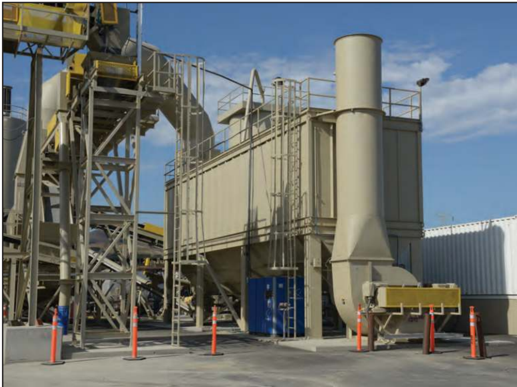
A 95,893 CFM Pulse Jet baghouse controls particulate matter by filtering the plant's exhaust through fabric filters before it enters air space.
