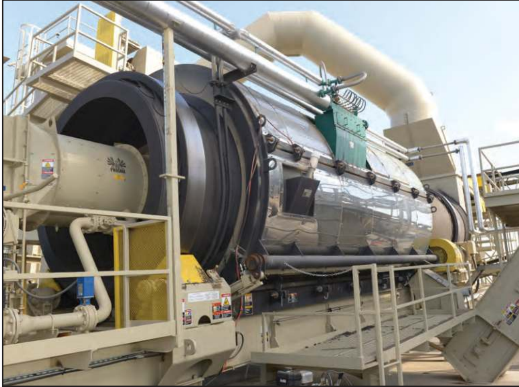
DeSilva Gates installed a 9 ft (2.74 m) Astec Double Barrel® drum mixer with warm mix system.
