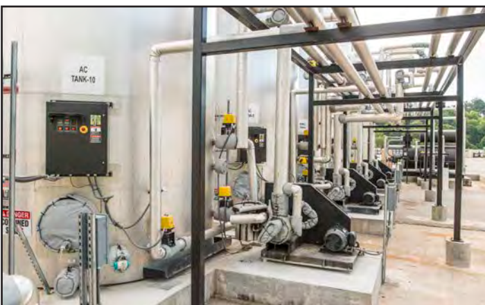
Overhead pipe routing allows easy access to other components. Hot oil piping is sized for fast heating. Unfortunately, we see many plants where these important features were overlooked. If you want it done right, let us design and install your piping.
