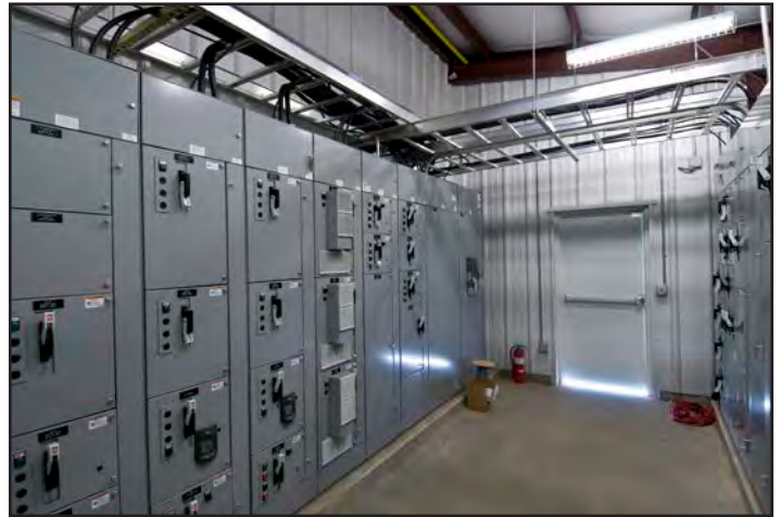
The motor control center centralizes all electrical power for the terminal and for the motor controls. The controls are housed in racks and panels. Power is sub-divided into independent control sections based on the location of the equipment.
