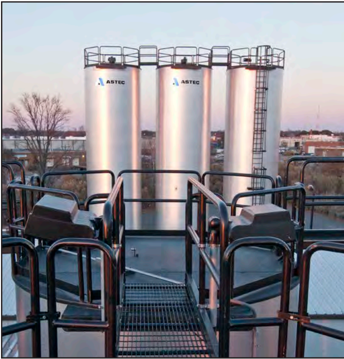
Heated 30,000 gallon tanks store base asphalt for emulsions. Two have mixers for PMAC. Interior walls have multiple coats of corrosion-resistant paint. Bridges interconnect the tanks.
