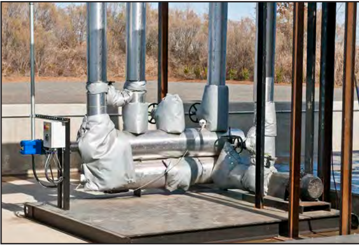
The warm oil skid blends some of the oil from the main supply line of the hot oil system with cooler oil. This lowers its temperature for pumps and asphalt piping heat-traced with hot oil.
