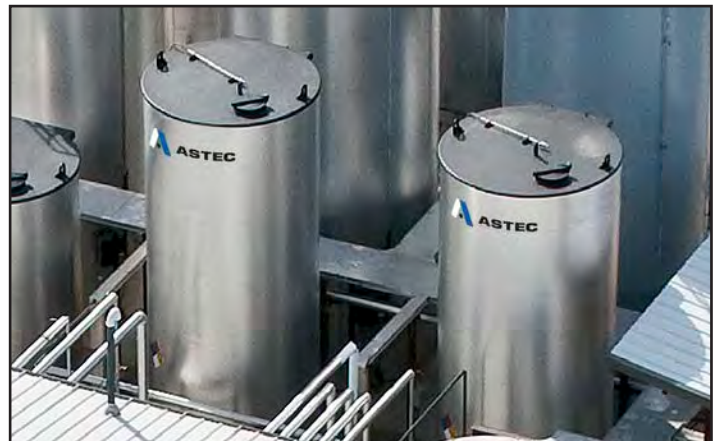
Two surfactant tanks, each with a capacity of 8,500 gallons. The tanks are insulated and heated electrically. They have pressure transmitters for level indications and have sampling valves.
