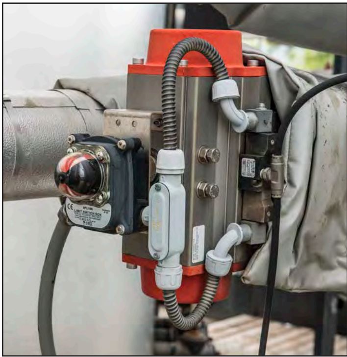
Actuated valves in asphalt piping are controlled by PLC. Valves and piping may be either jacketed and heated by hot oil or heat traced.
