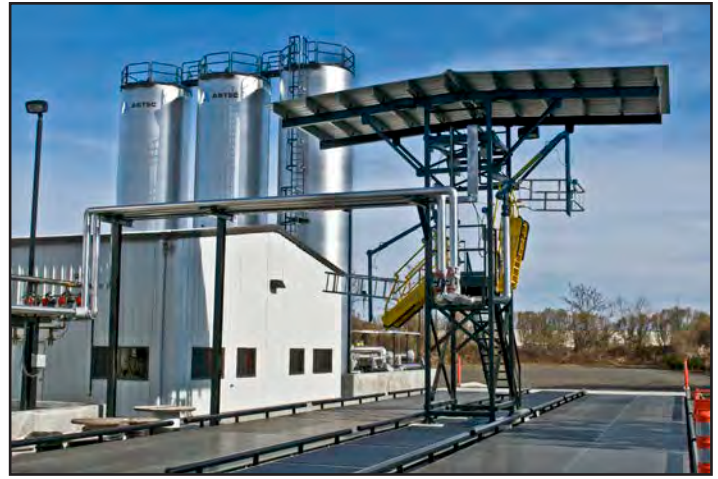
Plant personnel operate the load-out system to fill two tanker trucks simultaneously. Key features are PLC controls, two truck scales, loading arms, overflow protection and two walkout bridges with fall protection.
