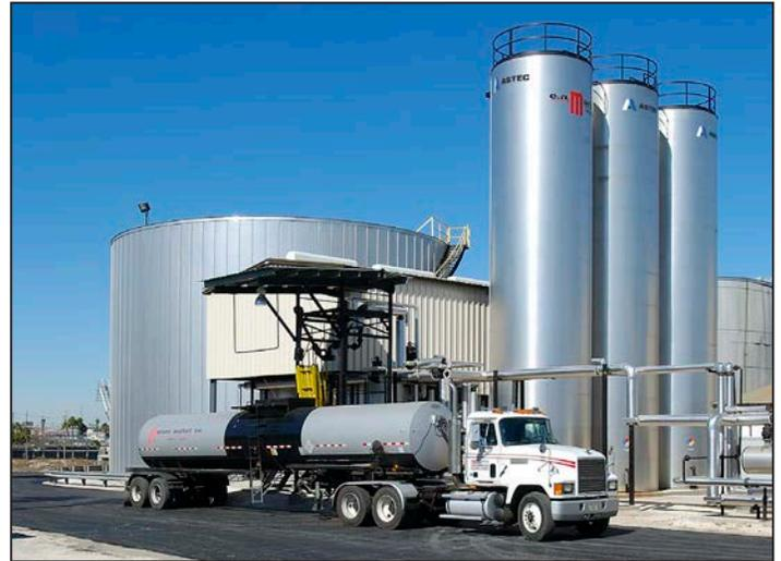
The three vertical tanks shown here are for polymer-asphalt storage. They are heated, insulated, and have mixers. Each tank holds 35,000 gallons.
