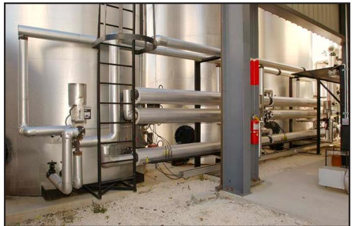
Astec normally pre-pipes the blending system at our factory using jigs for critical fits. This significantly reduces piping errors, speeds up field installation and reduces field re-works.
