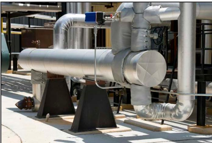
A booster heat exchanger may be required to increase the temperature required for blending.
