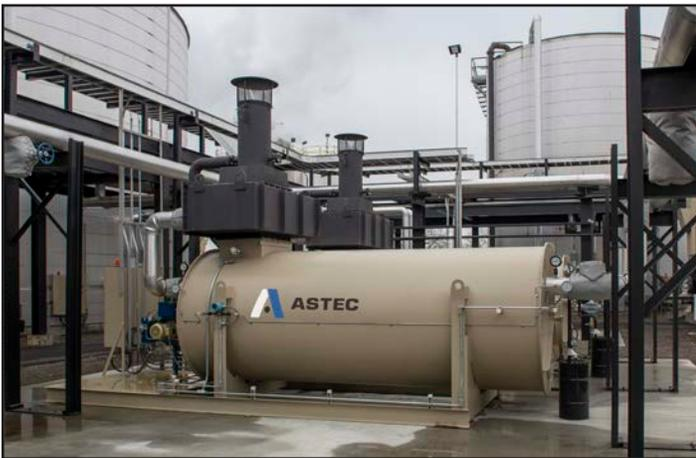
Heat for the polymer blending system is usually provided by the thermal fluid heater that heats asphalt storage tanks and other components at the terminal.
