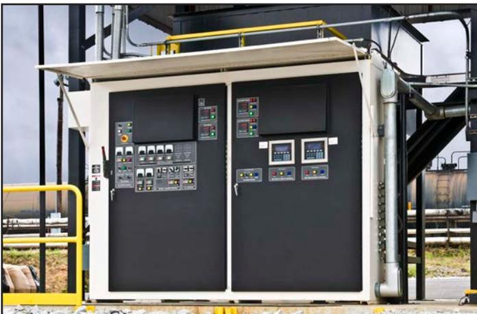
The main control panel for an early Heatec polymer system at an asphalt terminal. The operator initiates the blending process using controls on this panel. A PLC in the panel sequences the operations. Fiber-optic wiring, which is not affected by lightning strikes, can be used to interconnect panels in the system. Some of the controls on this panel are now replaced by a conventional desktop computer like the one shown above.
